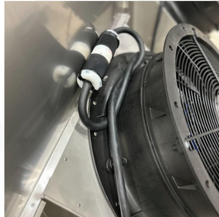
Fig. II.C.2.1 Male and Female plugs locked together
